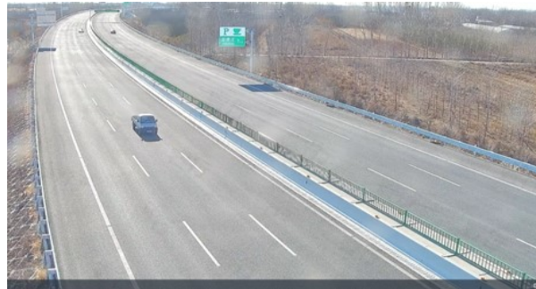
Figure 3. Expressway photo information.
