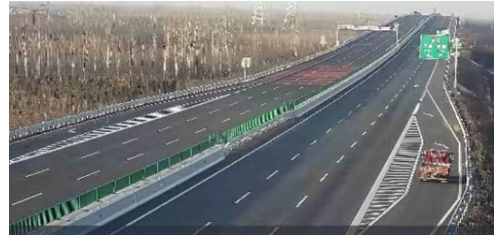
Figure 8. Emergency parking zones scene.
